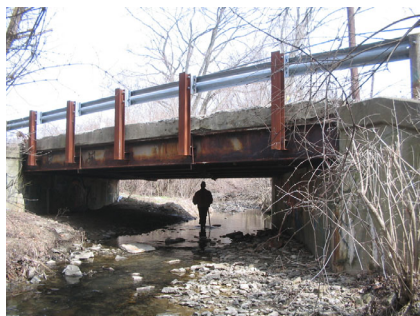
ELEVATION LOOKING EAST.
