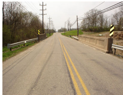
ENDVIEW LOOKING WEST.
