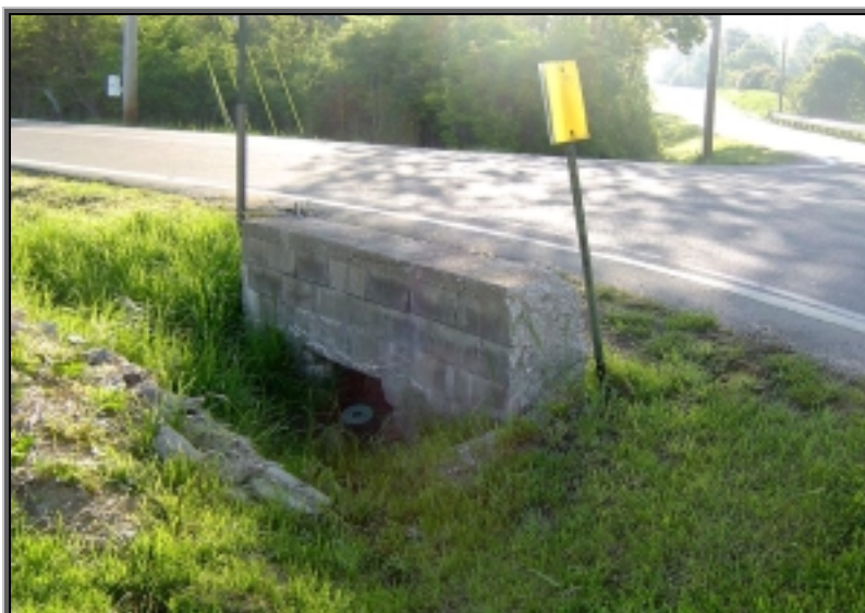
Bunker Hill Woods Road Culvert #01.131
