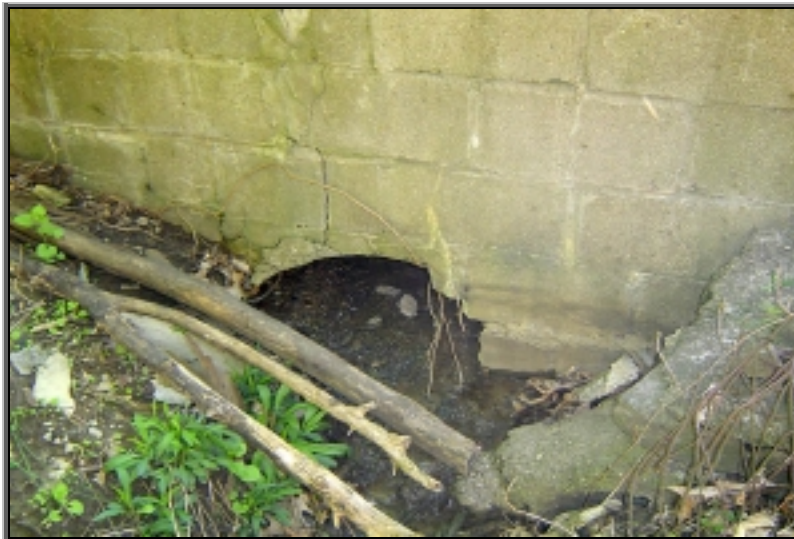
State Road Culvert #02.203
