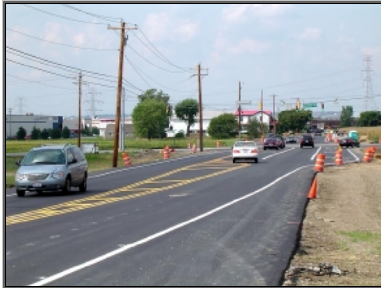
Intersection in 2006 during first phase of improvements.
