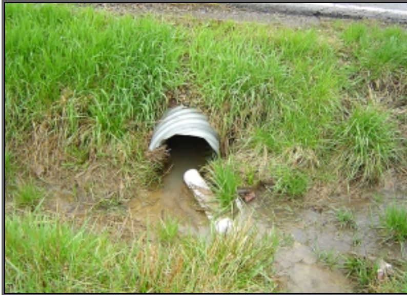
Stillwell Road Culvert #02.787
