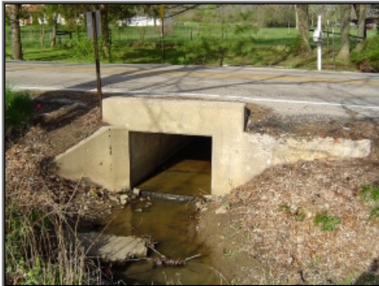
Eaton Road Culvert #07.208
