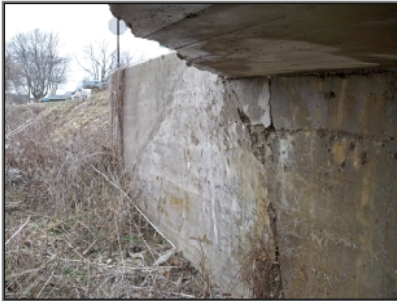
Hamilton Eaton Road Culvert #06.562
