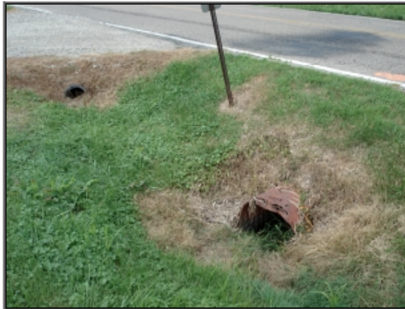
Fairfield Road Culvert #01.180
