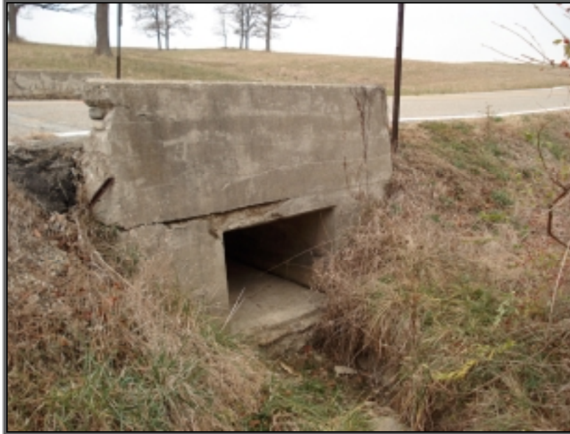
Springfield Road Culvert #01.658
