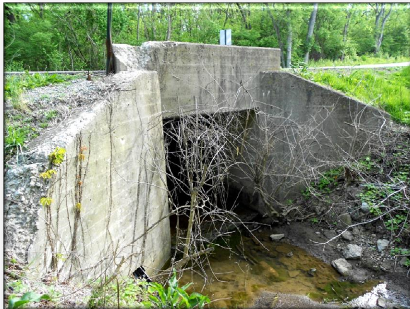
Hamilton Mason Road Culvert #05.452
