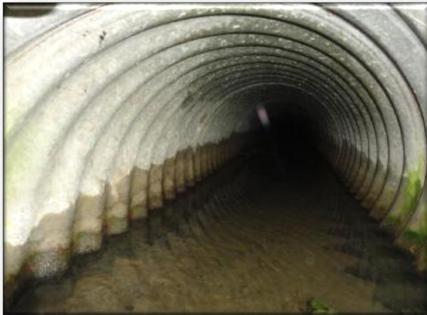
Middletown Germantown Road Culvert #01.203
