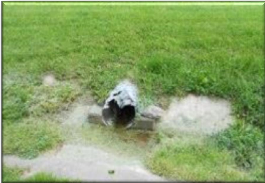
Brown Road Culvert #01.886
