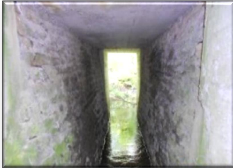
Hamilton Mason Road Culvert #05.422
