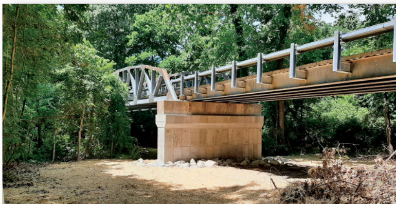
Buckley Road Bridge #3.90 Pier Rehabilitation Total Construction Cost: $235,188 Funding: BCEO
