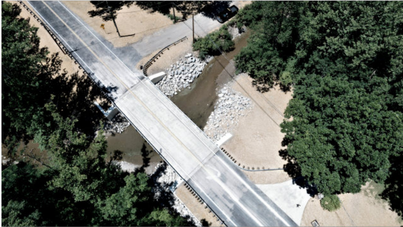
Bonham Road Bridge #1.603 Design-Build Bridge Replacement
