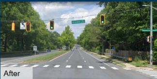
Signal changes at Shady Grove Rd & Briardale Rd with exclusive red turn phasing and backplates to address failure to yield crashes.
